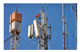
Figure 3. Base transceiver station (BTS)
